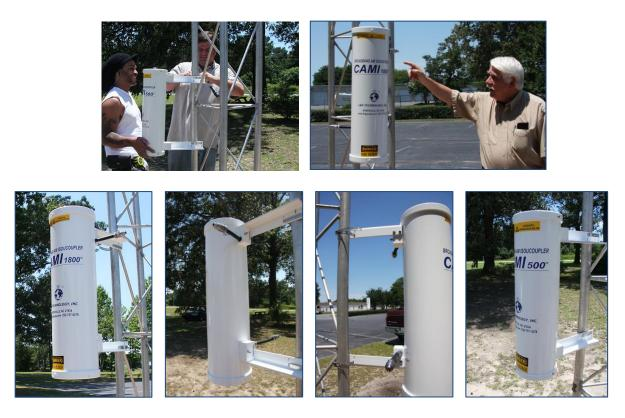
Note that these **CAMI**<sup>™</sup> models come with an insulated mounting kit. The pictures show the typical mounting on tower. The same kit enables mounting on a separate post, or horizontally under an ice bridge. Although mounting options are flexible, the following considerations should be kept in mind:
